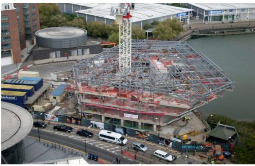
The structural frame of Canada Water Library is close to completion and the latest progress image shows the lattice effect of the steel roof trusses. The overall form of the new building is clearly apparent, revealing the striking design and steeply raking angles of the structure over the Canada Water Basin.
