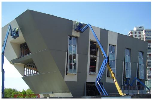
Mobile Elevating Work Platforms or MEWPS are being used extensively as we reach the latter stages of the project to build Canada Water Library. These platforms enable our specialist teams to safely apply the high performance waterproof membrane and mesh rainscreen cladding to the building's façade.
