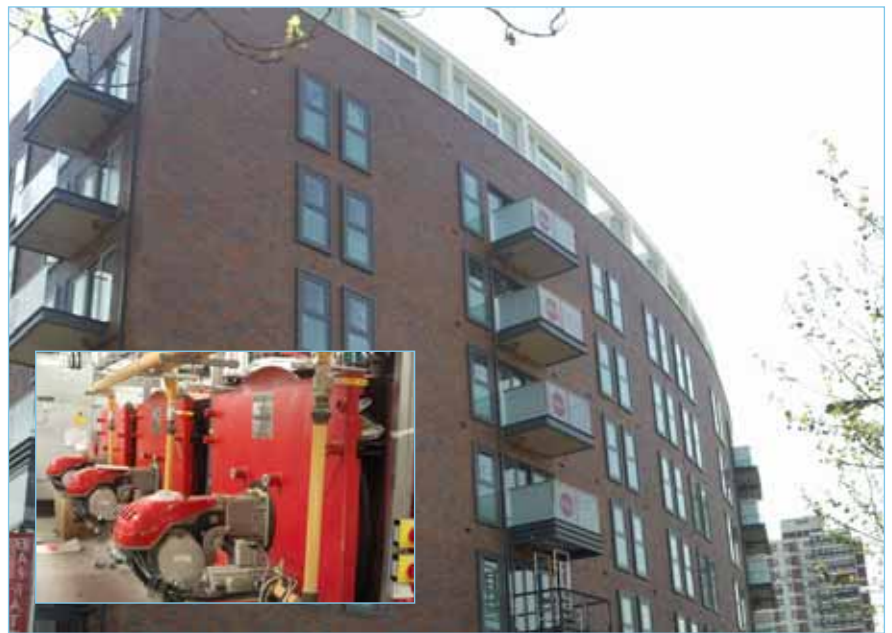
Site B2 nearing final completion
