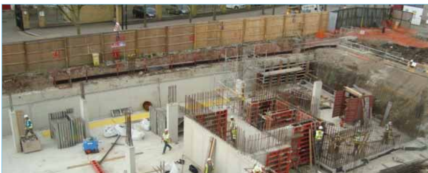
Site A1 works well underway
